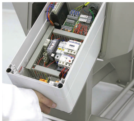
Sliding electrical box for easy access
